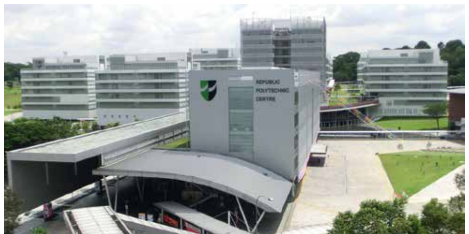
Republic Polytechnic Center, Singapore, 2006 Architects Fumihiko Maki, DP Architects; Sealed with Sikasil® WS-605 S, after >5 years no signs of streaking effect
