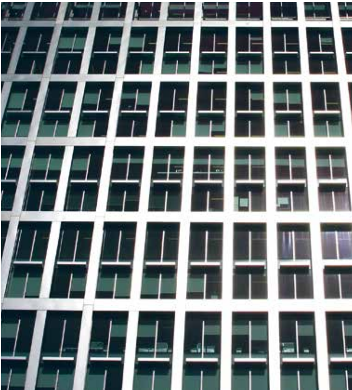
5 Aldermanbury Square, London, 2005 Architects Eric Parry Architects; Facade Lindner-Schmidlin UK
