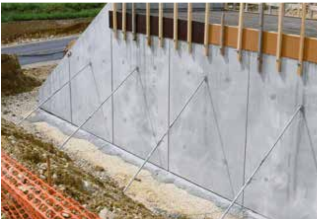
Precast concrete elements
