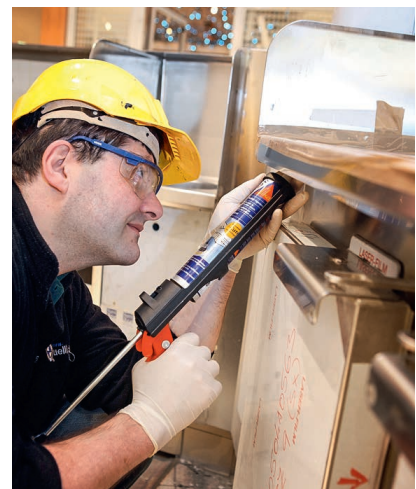
Fig. 9 Application of Sikaflex®-291i
