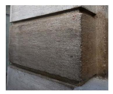
After all these tests, Sika systems were approved. Marble surfaces would be coated not only with **Sikagard®-790 All-in-One Protect**, but with **Sikagard®-850 AG** because of the high protection level that the product ensured from vandalisms (posters and graffiti).
