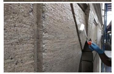
Application of the second layer was performed 2 to 3 hours after the first coating (touch dry). Finally, after finishing the application, graffiti spray was again applied on the **Sikagard®-850 AG** coating to evaluate its performance. After a few hours, it was cleaned by cold-water low pressure water, proving again its exceptional characteristics.
