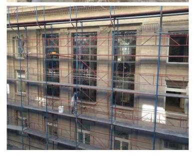
7 days afterwards (complete curing of Sikagard®-730 Concrete Protect Plus), Sikagard®-907 W was applied, which works parallel as a sealing resin and surface stabilizer for friable substrates. The product was applied in 2 to 3 coats with roller and brush in the joints (wet-to-wet method), depending on the condition of the coating.
