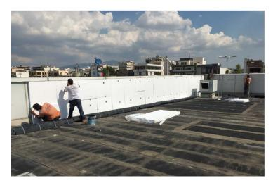
**Sikaplan® TM-15** membrane was mechanically fastened using auxiliary products for linear and point support.
