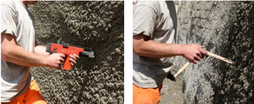
Fig. 8.4 / 8.5: Penetration of young sprayed concrete with studs using a Hilti DX 450-SCT (left) and measurement of the stud protrusion for the determination of the penetration (right)
