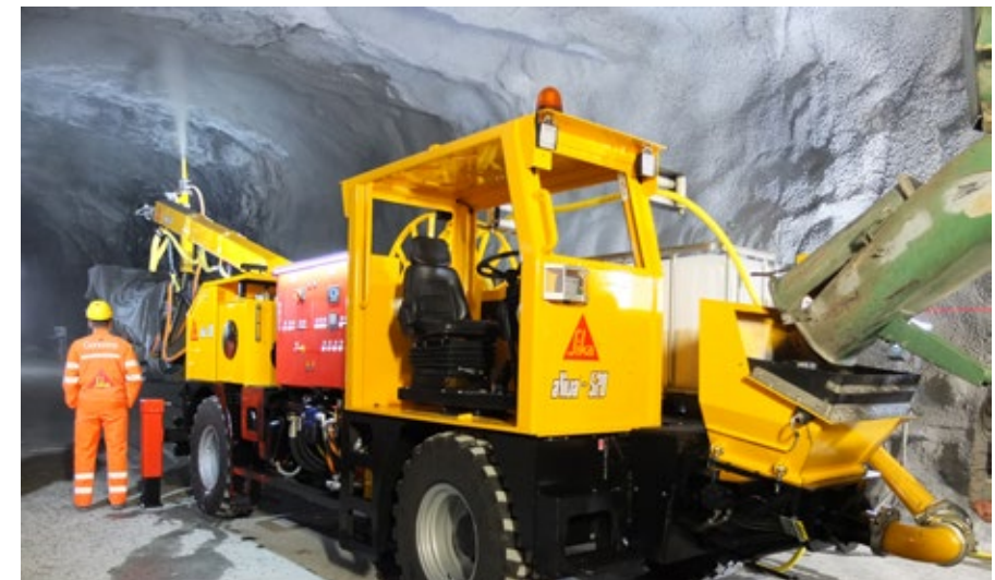
Fig 1.3: Shotcrete application, high degree of mechanization
