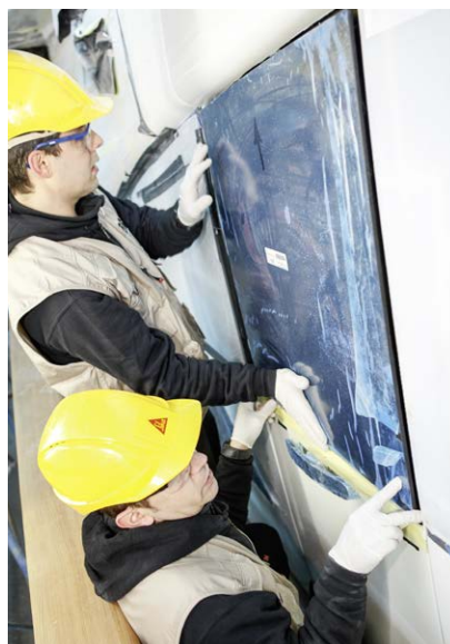
Fig. 7 The window is fitted
