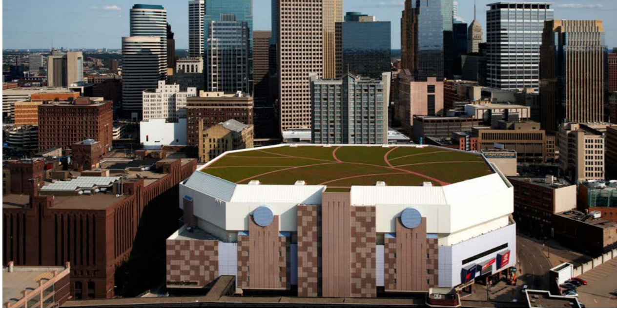
Target Center sports and entertainment arena, Minneapolis, USA
