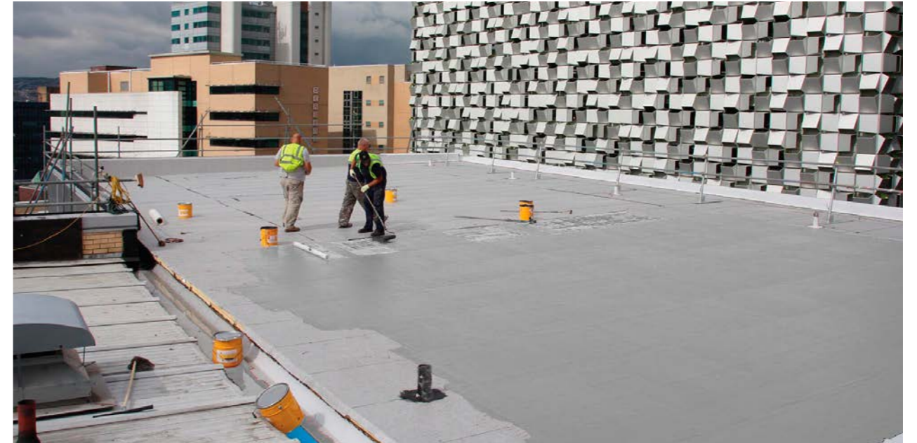
Liquid-applied membrane application, Hallam University, Sheffield, UK
