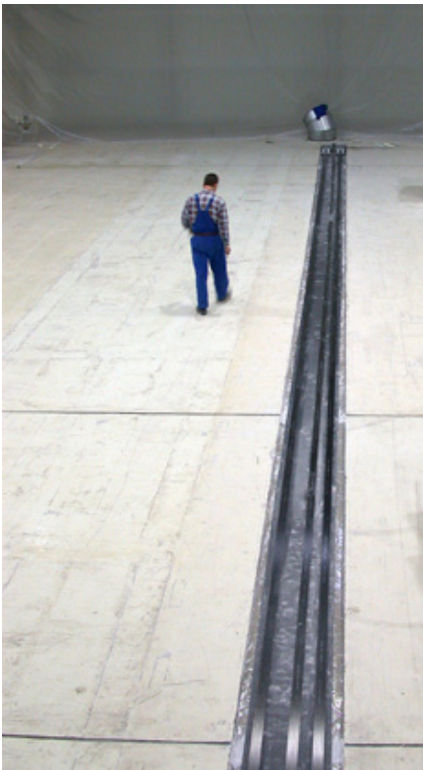
The longest post-tensioned CFRP-plates ever installed
