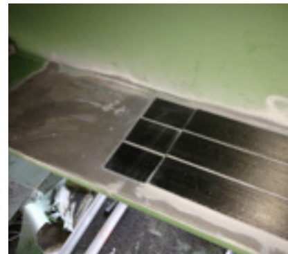
Two layers of Sika CarboDur®
