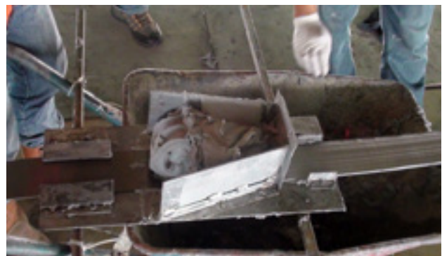
Coating of CarboDur® plates with Sikagard®
