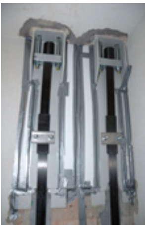
Anchorage of Sika CarboStress System
