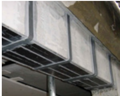
BEAM STRENGTHENING
