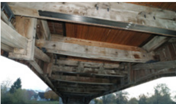
CarboDur® strengthened crossbeam
