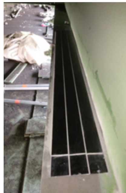
Two layers of Sika CarboDur®
