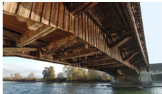
Bottom view of strengthening system
