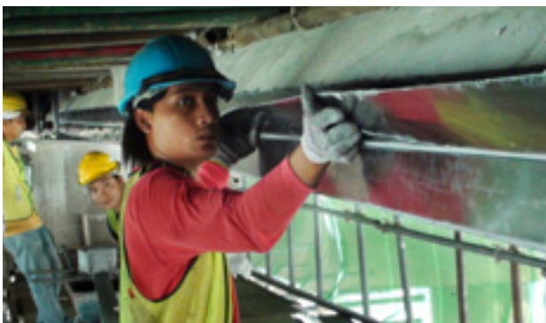
Installation CarboDur®
