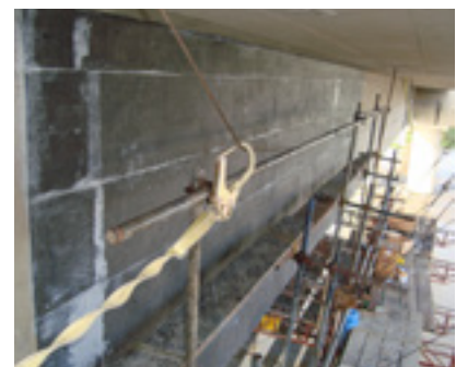
Strengthening with SikaWrap®
