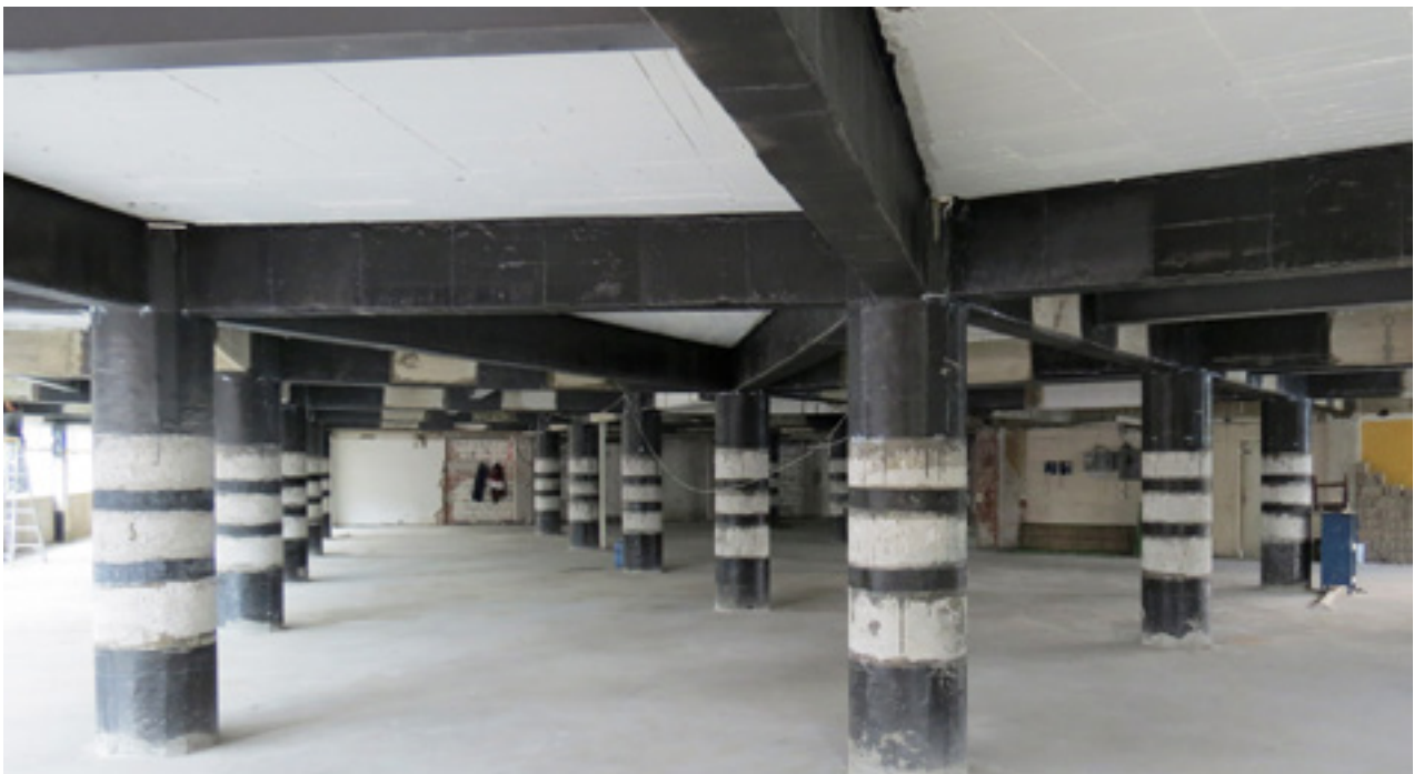
Beams and columns strengthened with SikaWrap®
