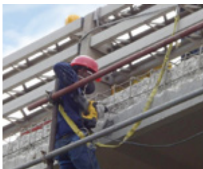
Substrate preparation
