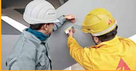
CORROSION AND FIRE PROTECTION
