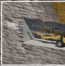
Control of over-blast
