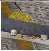
Cavity and void filling
