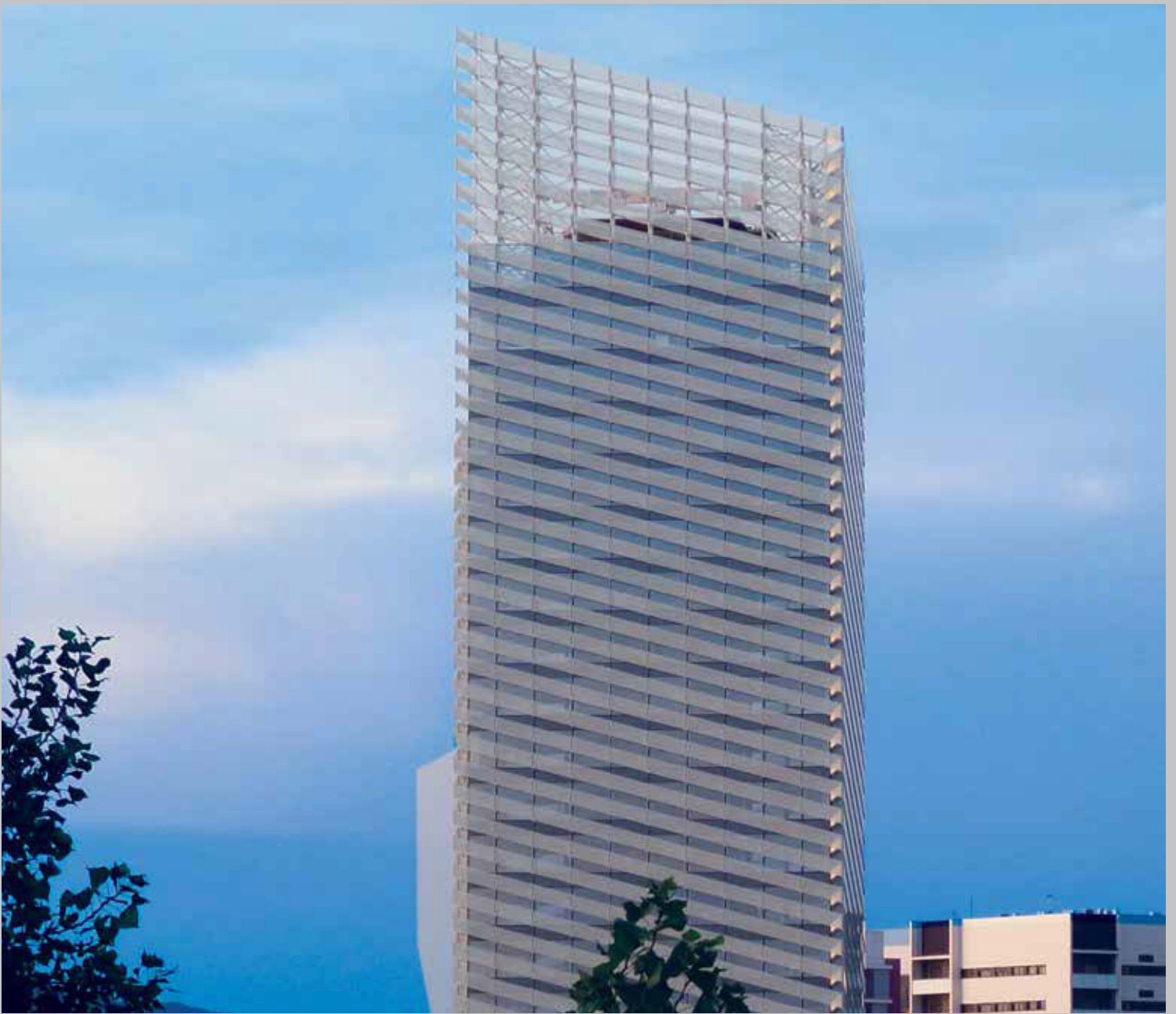
Torre Puig, Barcelona, bonded with Sikasil® SG-550 and Sikasil® IG-25 HM Plus
