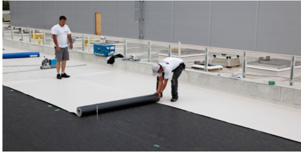
Application of roofing membrane above the Sika® RCS Glass Fleece.
