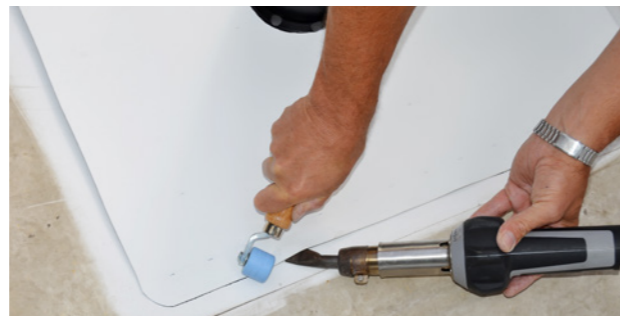
Preparation of appropriate roofing membrane patch, hot air welded.
