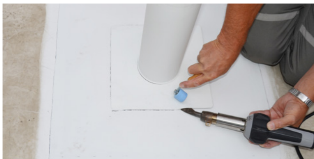
Sealing of the Sarnafil® Control Pipe and subsequent seam inspection.
