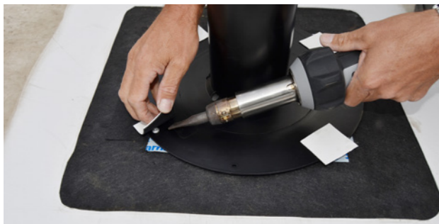
Fixing the RCS Cable Access Duct with base plate to the substrate. Covering the screw head with a piece of membrane.
