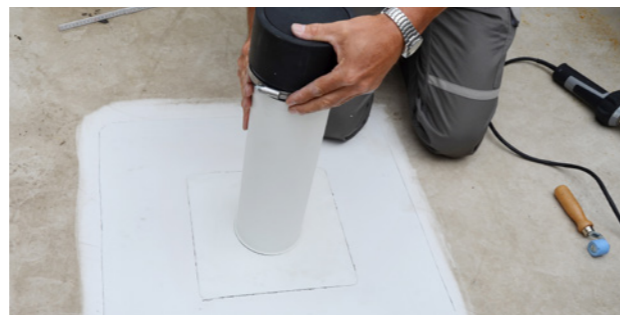
Finished Sarnafil® T RCS set.
